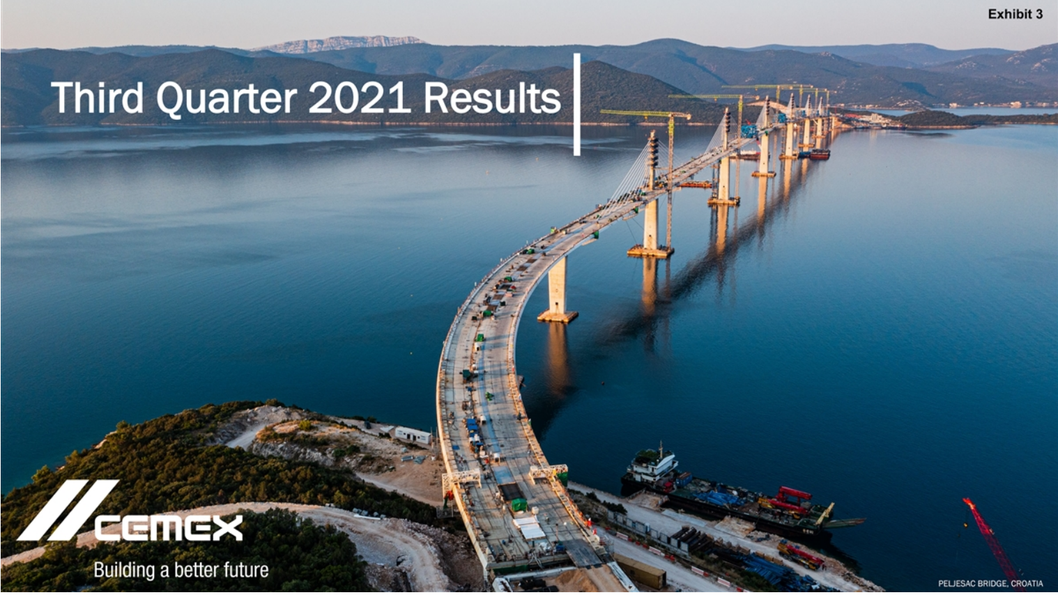
PELJESAC BRIDGE, CROATIA
