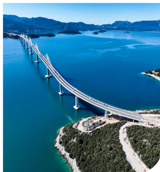
Pelješac Bridge, Pelješac, Croatia Built with Vertua Concrete, part of our Vertua family of sustainable products
