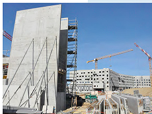
LA CROIX DU SUD CLINIC CONSTRUCTION PROJECT IN TOULOUSE, FRANCE
