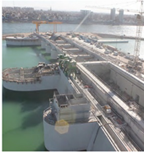
ASSIUT BARRAGE AND HYDRO-POWER PLANT, EGYPT
