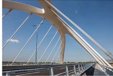
NELSON MANDELA BRIDGE, BARCELONA, SPAIN
