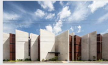
AFFORDABLE HOUSING Salvatierra 150. Mérida, Mexico
