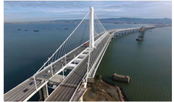
San Francisco Bay Bridge, USA
