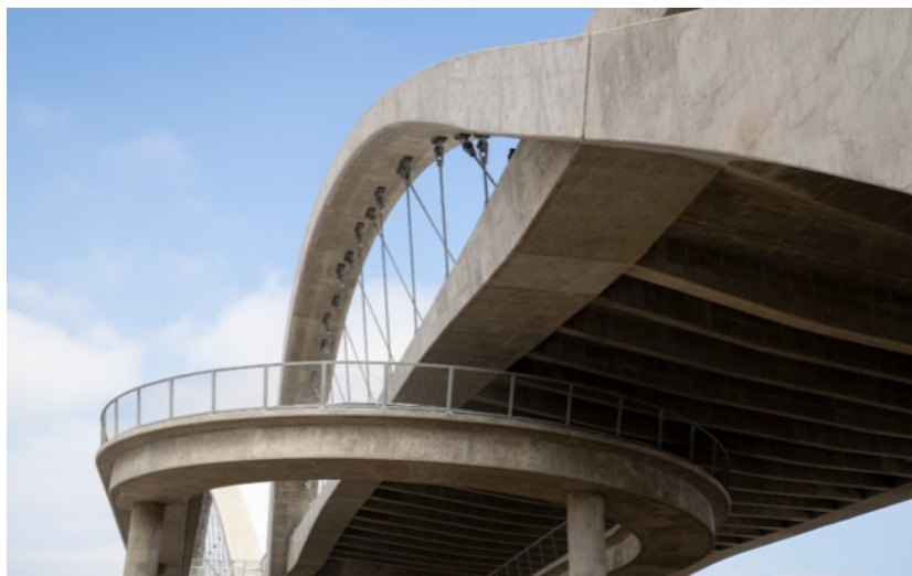
Sixth Street Viaduct, Los Angeles, United States
