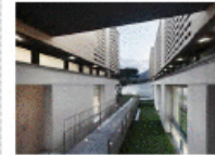
SPECIAL PRIZE Sustainable Building: Oak House School Barcelona, Spain
