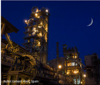
Buhil Cement Plant, Spain
