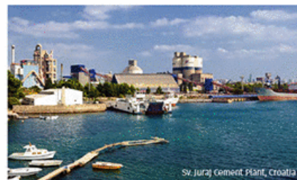
Sv. Juraj Cement Plant, Croatia
