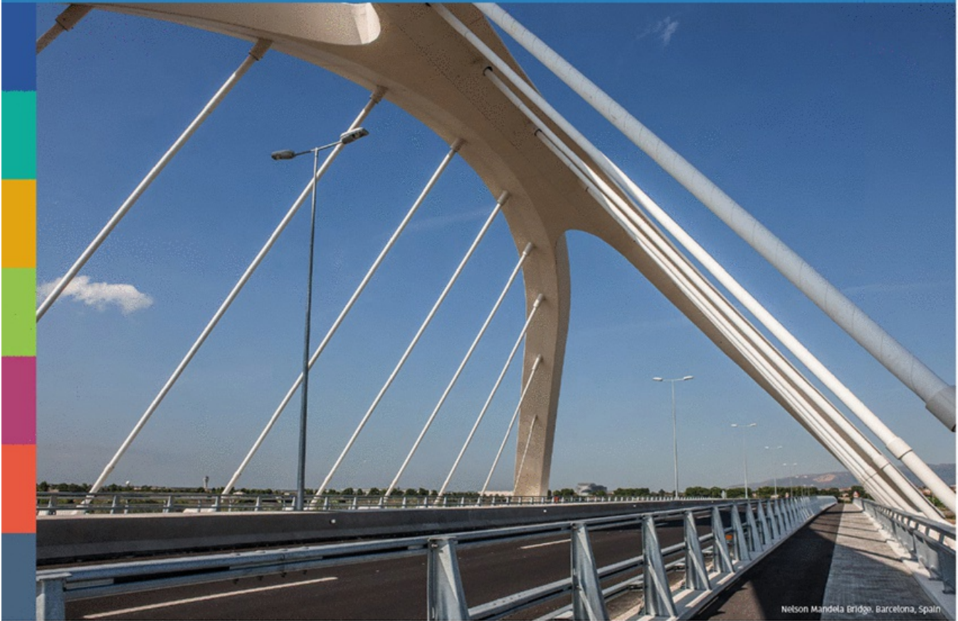
Nelson Mandela Bridge, Barcelona, Spain
