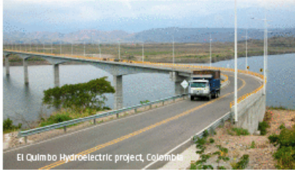
El Quimbo Hydroelectric project, Colombia
