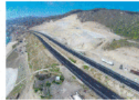
Infrastructure: Restitution of Embankment in Tijuana-Ensenada Highway at KM 93 Ensenada, Mexico
