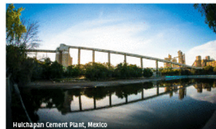
Hulchapan Cement Plant, Mexico
