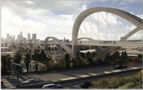
Los Angeles, CA – Sixth Street Viaduct
