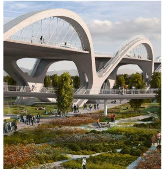
6th Street Viaduct, Los Angeles, USA Built with Vertua concrete, part of our Vertua family of sustainable products
