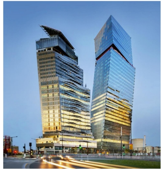
Duo Towers, Paris, France Built with Vertua Concrete, part of our Vertua family of sustainable products Picture by Jad Sylva Photography
